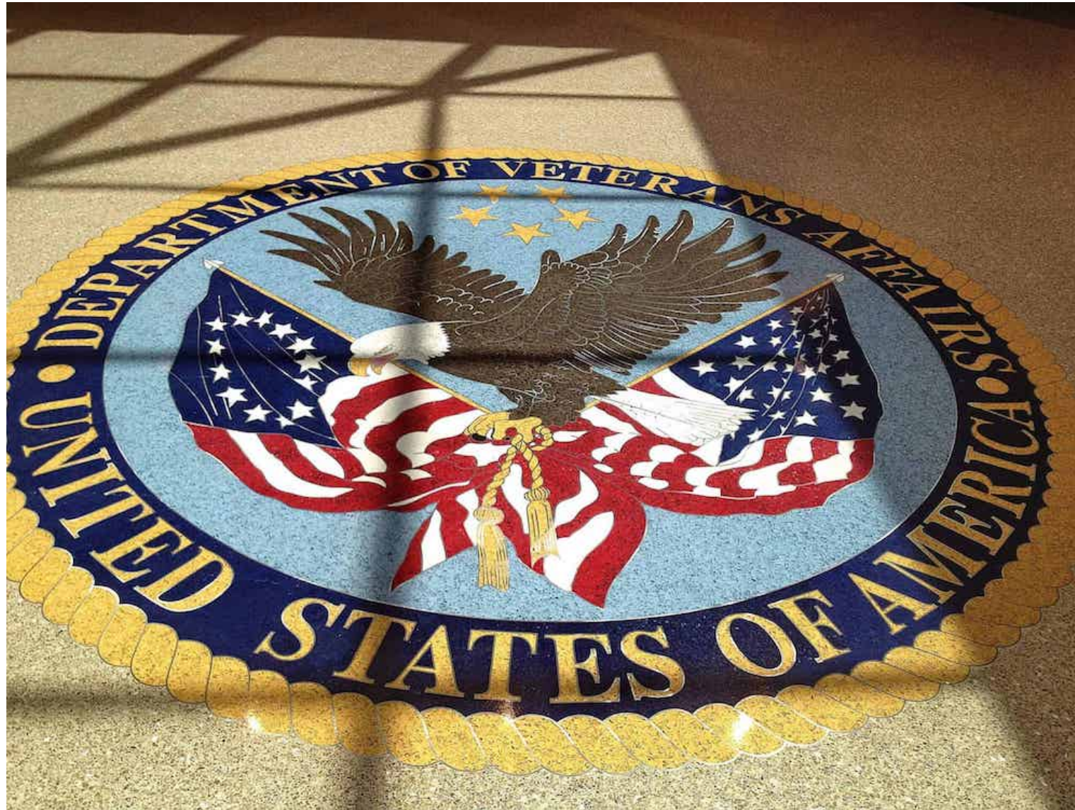
A LOBBY - TERRAZZO EPOXY FLOOR DESIGN
